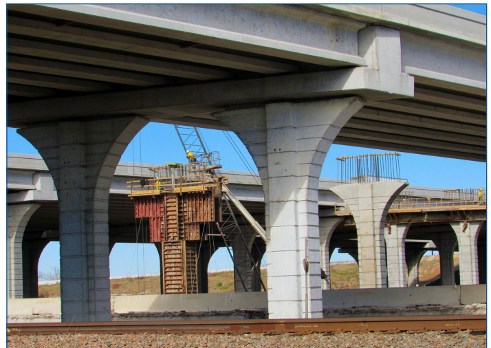
I-69 expansion nears completion in Rosenberg, Texas
